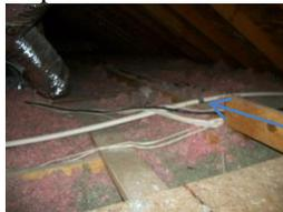
Drain line should not slop up. Does not allow water to drain correctly
